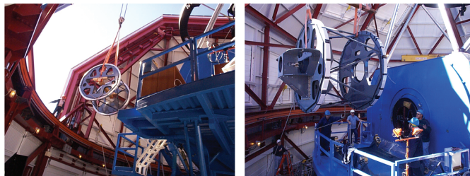
FIG. 37.— Left: In 2003 August, IMACS is raised from a palette outside the Magellan enclosure by the dome crane and lifted through the dome slit. Right: IMACS is positioned on the west Nasmyth platform.
